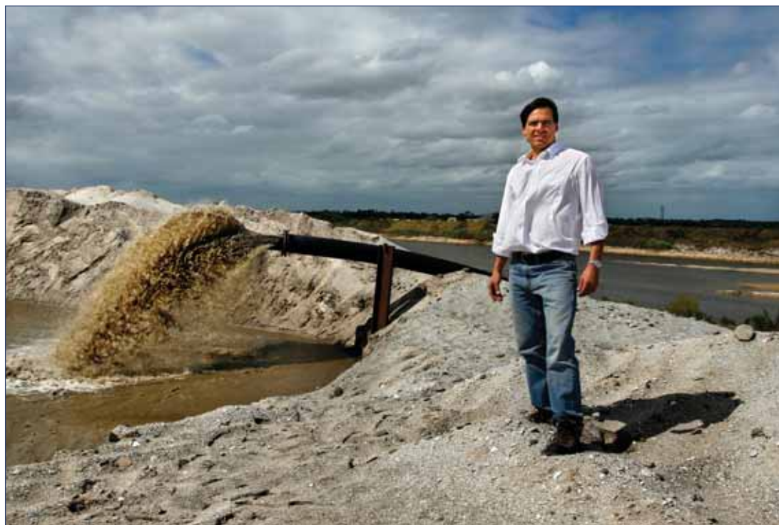
Real estate developer Stephen Smith, co-owner of Ranch Road Lake LLC, on the site of his sand mine with the dredge equipment that has already spewed out most of the sand needed for barrier island beach replenishment. Story on page 8 Photo: Tom McCarthy, Jr.
